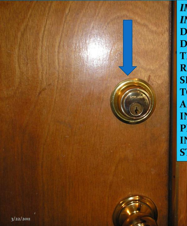
**IMPROPER LOCK INSTALLATION DOUBLE KEYED DEADBOLTS OR LOCK THAT WOULD REQUIRE A KEY OR SPECIAL EQUIPTMENT** TO OPEN ARE NOT **ALLOWED ON THE INSIDE OF THE** PROPERTY. **INSTALL THUMB TURN STYLE**
