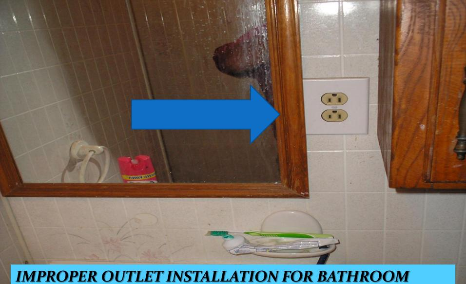
IMPROPER OUTLET INSTALLATION FOR BATHROOM OUTLETS IN THE BATHROOM MUST BE GROUND FAULT CIRCUIT INTERRPTOR PROTECTORED
