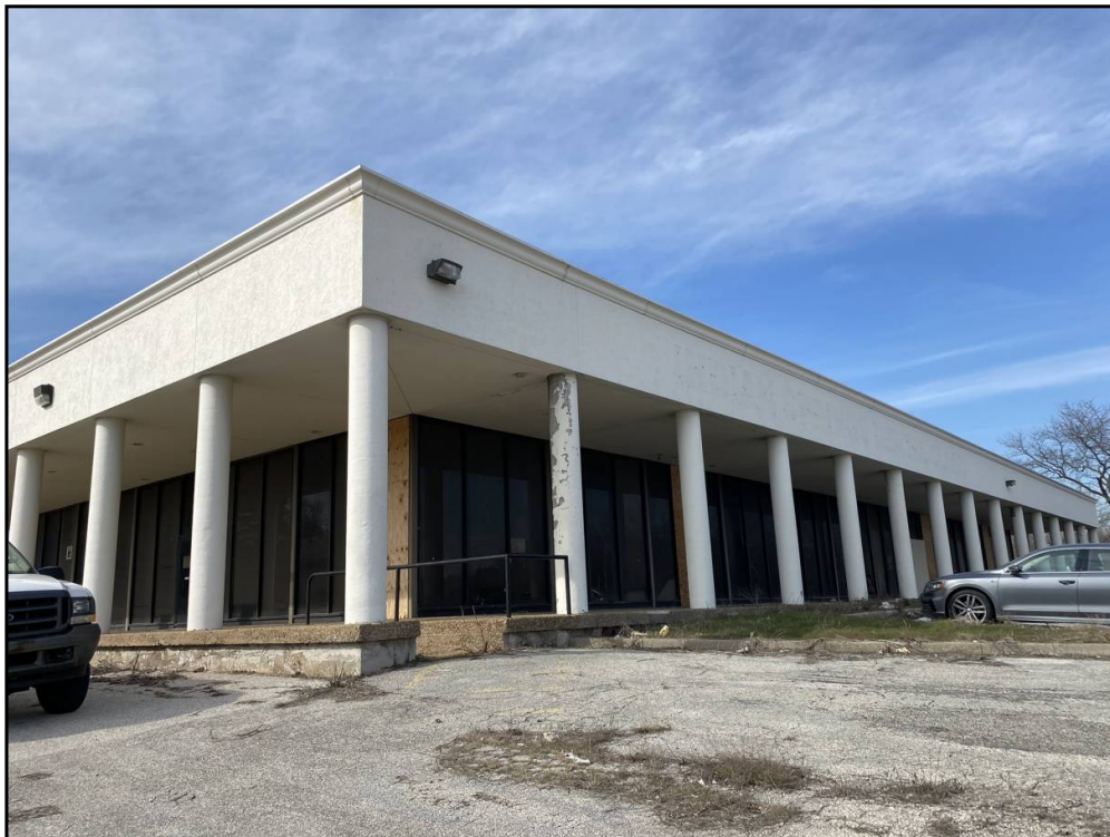
Northwest - View of unoccupied commercial structure on the northwest corner
