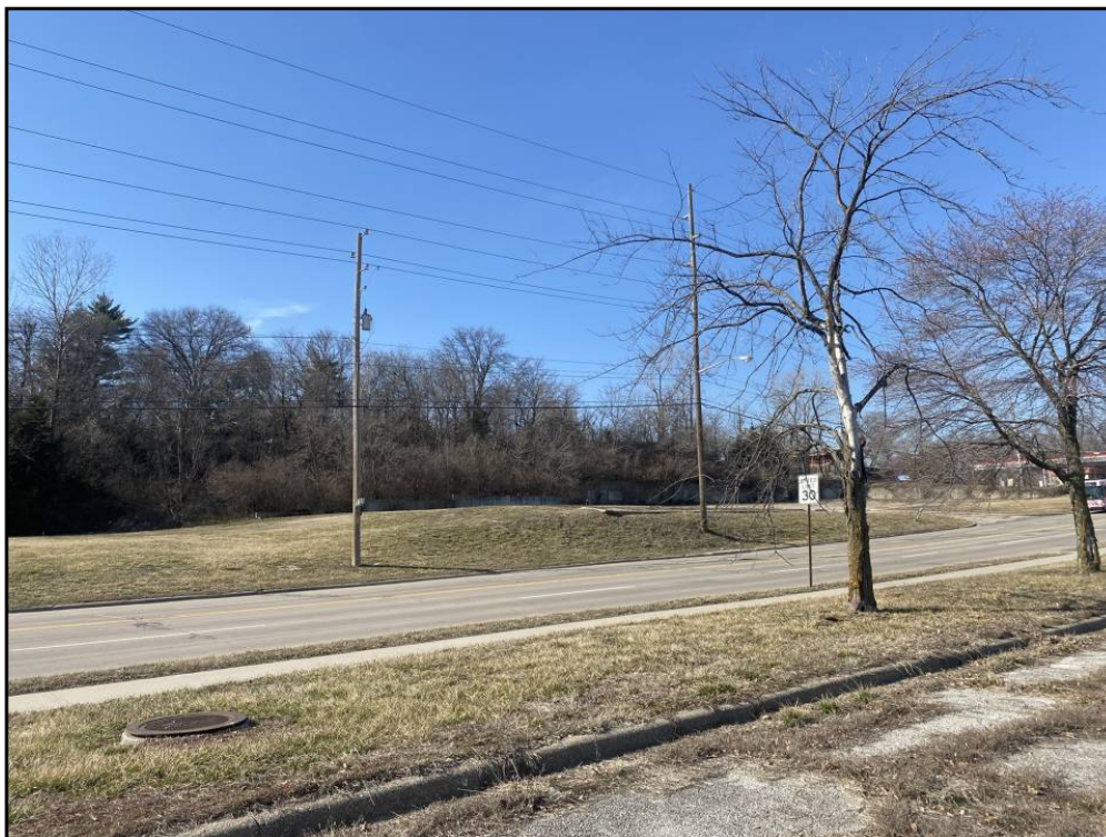
Northwest - View of west adjoining N 47th Street with vacant lots beyond
