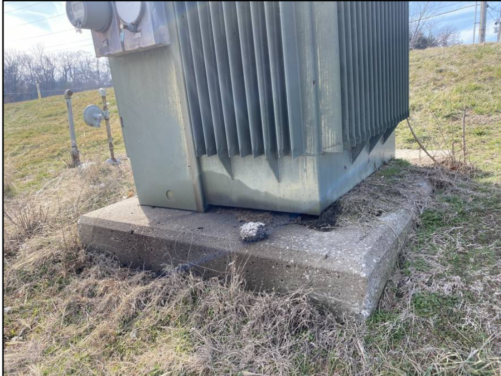
View of de minimis staining on non-PCB transformer
