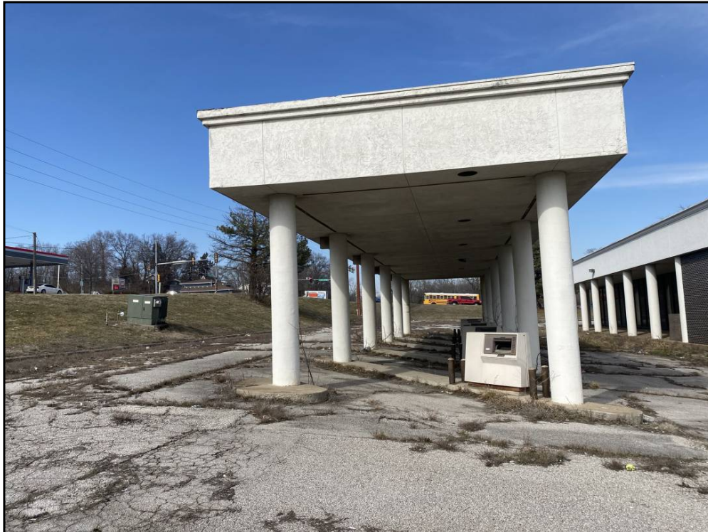
North - View of former bank service lanes on northwest corner
