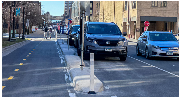
Doweled Concrete Curbs
